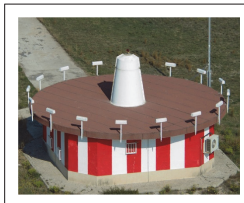
Figure 1. Station sol VOR.
